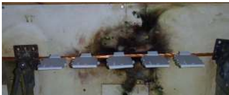
Figure 4-10: Mounting of PCS cards on down conductor
