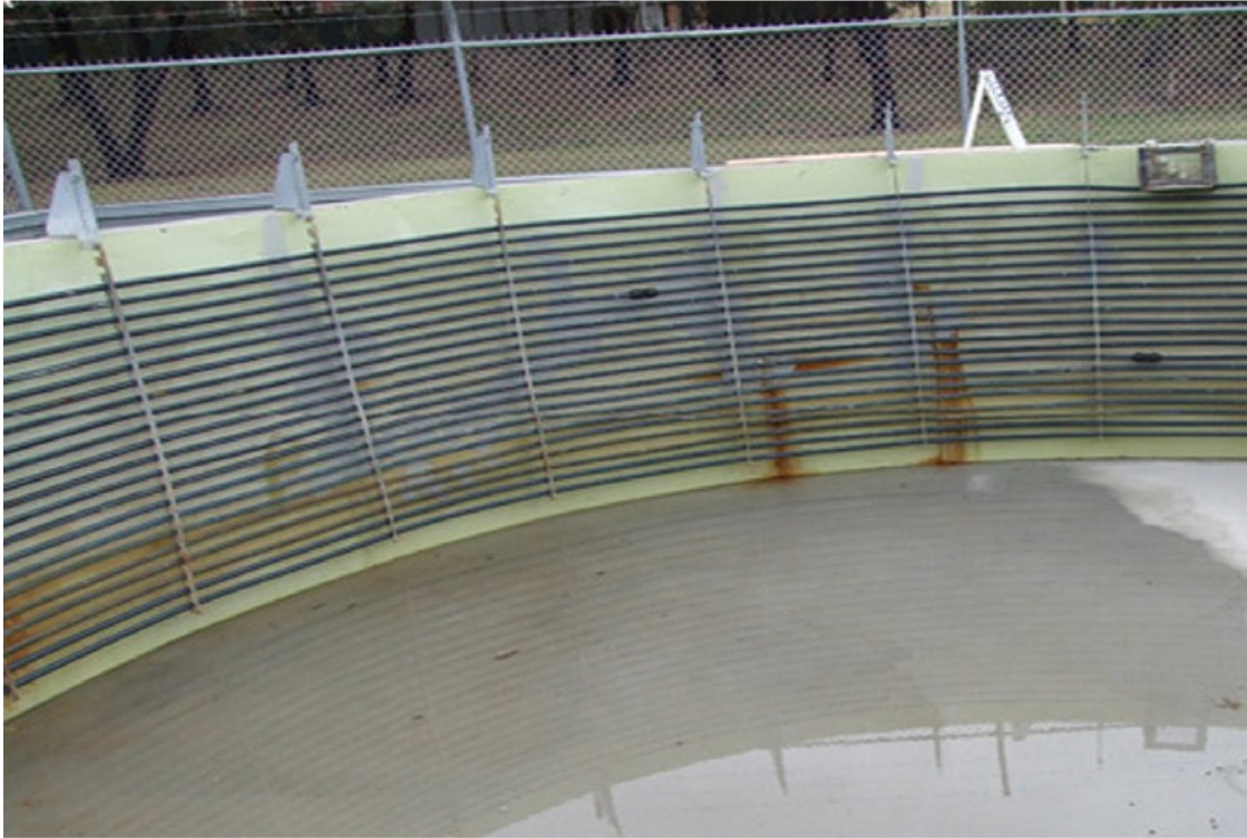
Figure 2.23 Inpond heat exchanger for gradient layer and LCZ (Leblanc et al, 2011).
