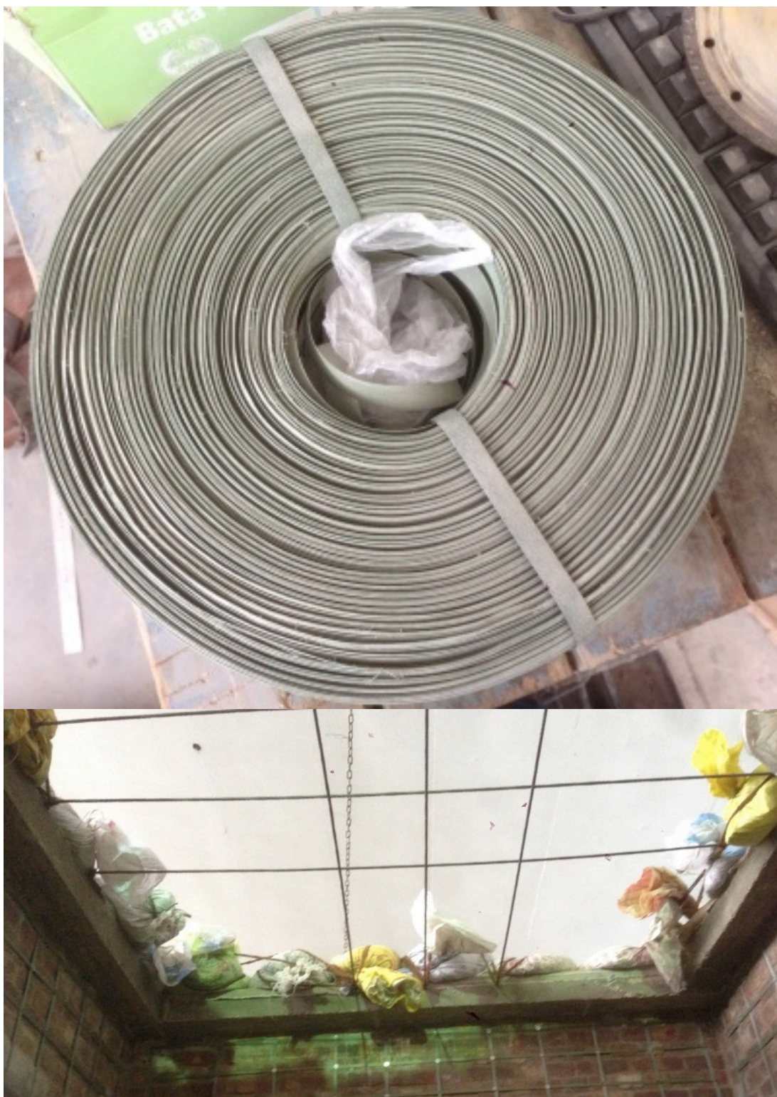
Figure 7.4: Typical roll of PP-band sold in the market ( top ), inside view of the roofing detail showing steel reinforcements connecting opposite beams ( bottom )
