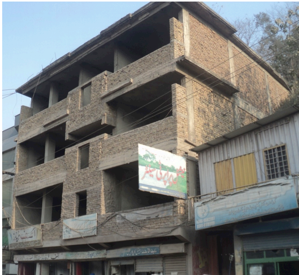
Figure 3.2: Structure with large openings in one direction and discontinuous RCC horizontal member
