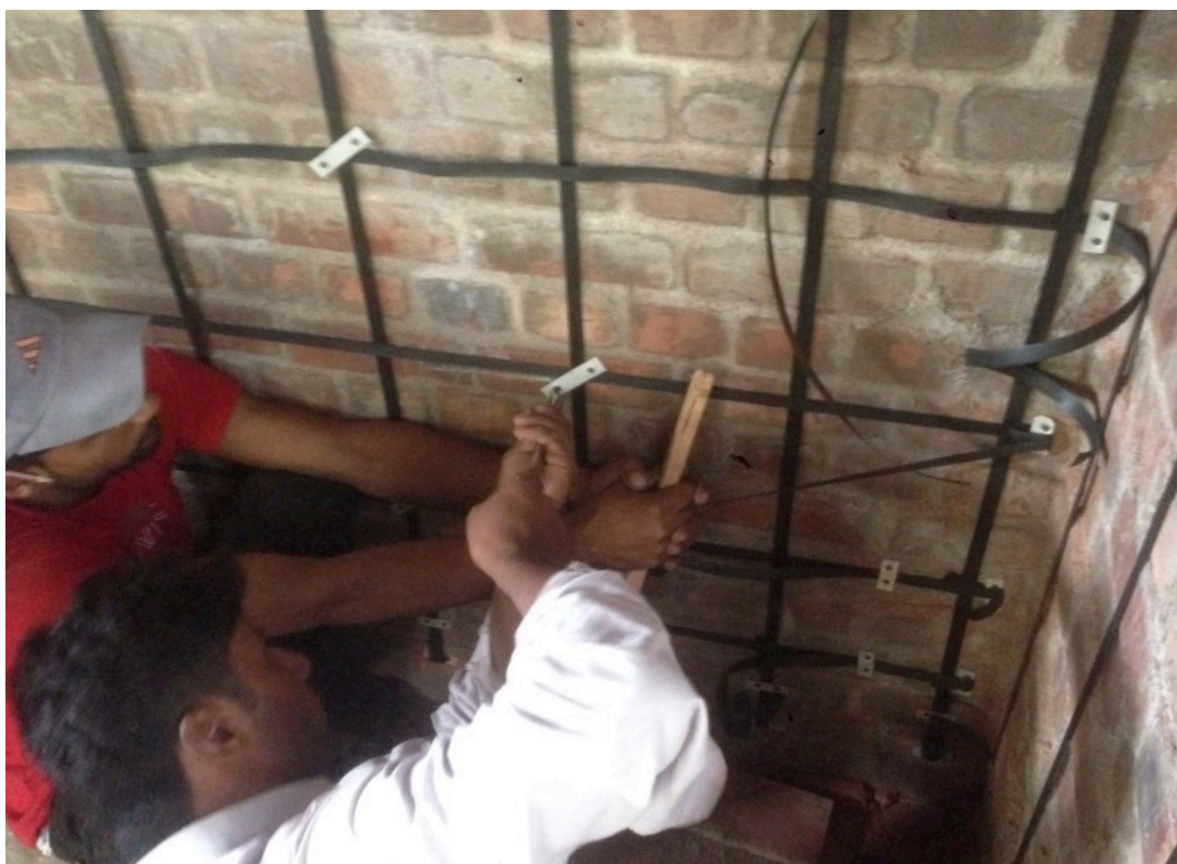
Figure 7.10: Applying tension in PP-bands to remove looseness before fixing Second end
