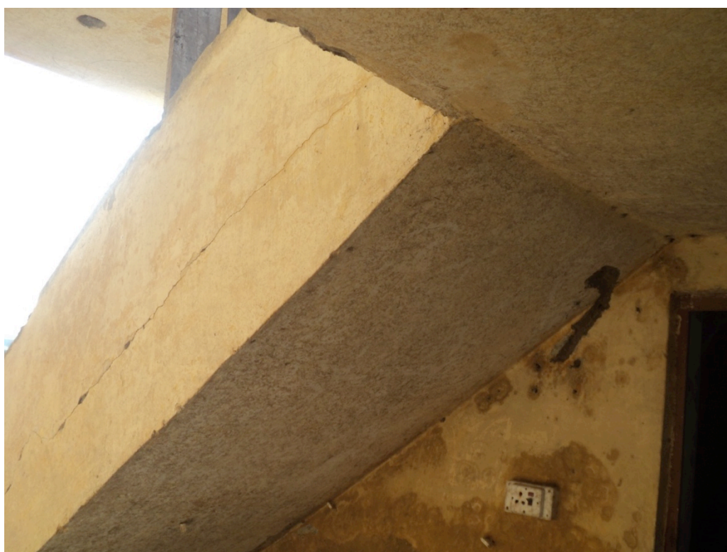
Figure 3.16: Stairs resting on the wall of structure
