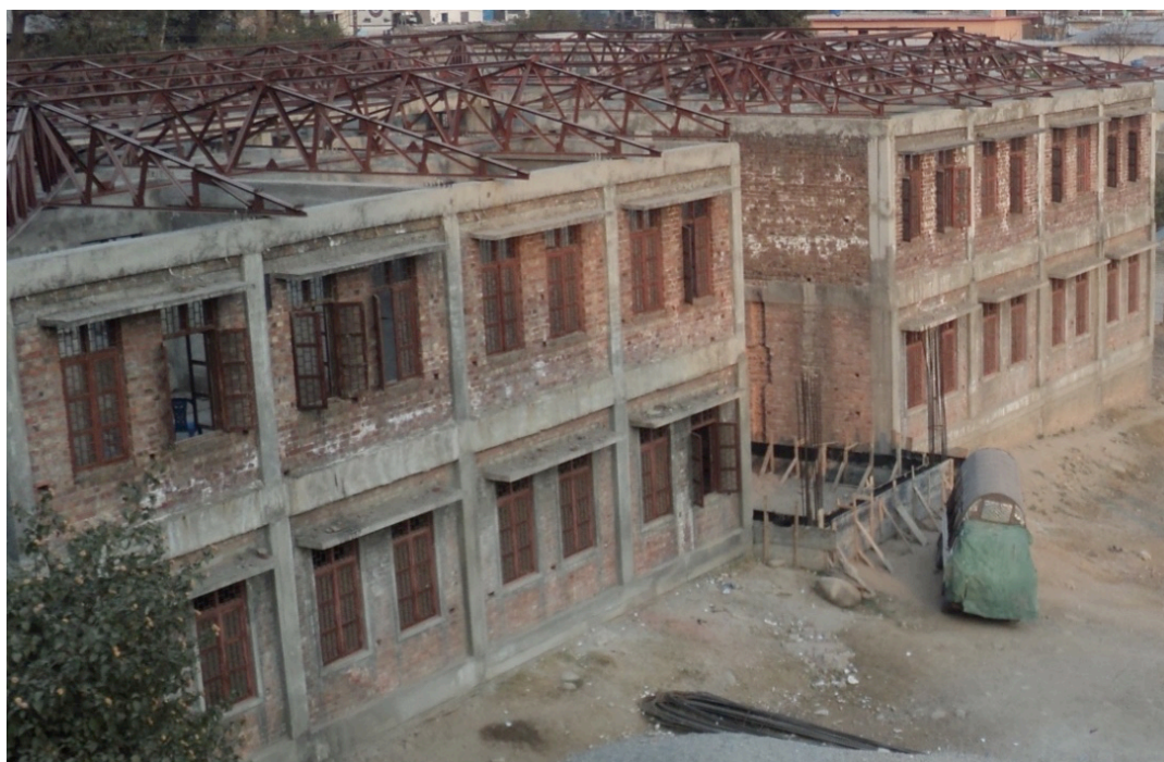
Figure 3.6: Government school building with proper confinements and lightweight steel roof
