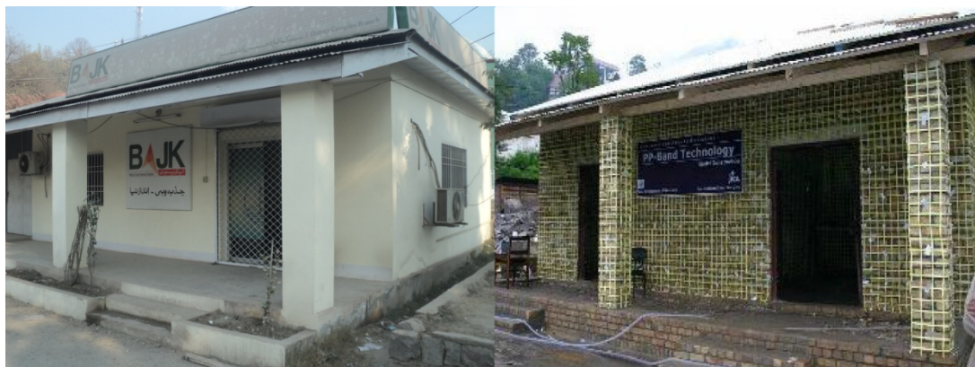
Figure 3.11: (Left) Structure in-use by local bank. (Right) PP-band mesh structure [73].
