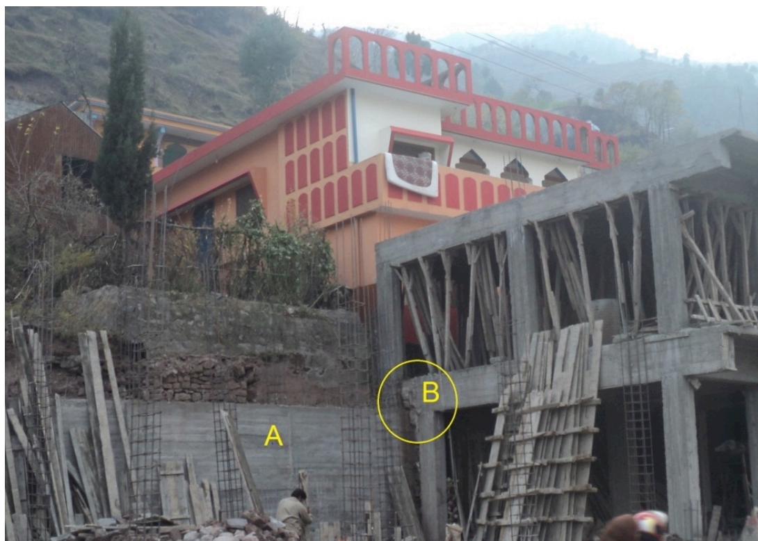
Figure 3.8: Back wall against hill slope constructed of RCC
