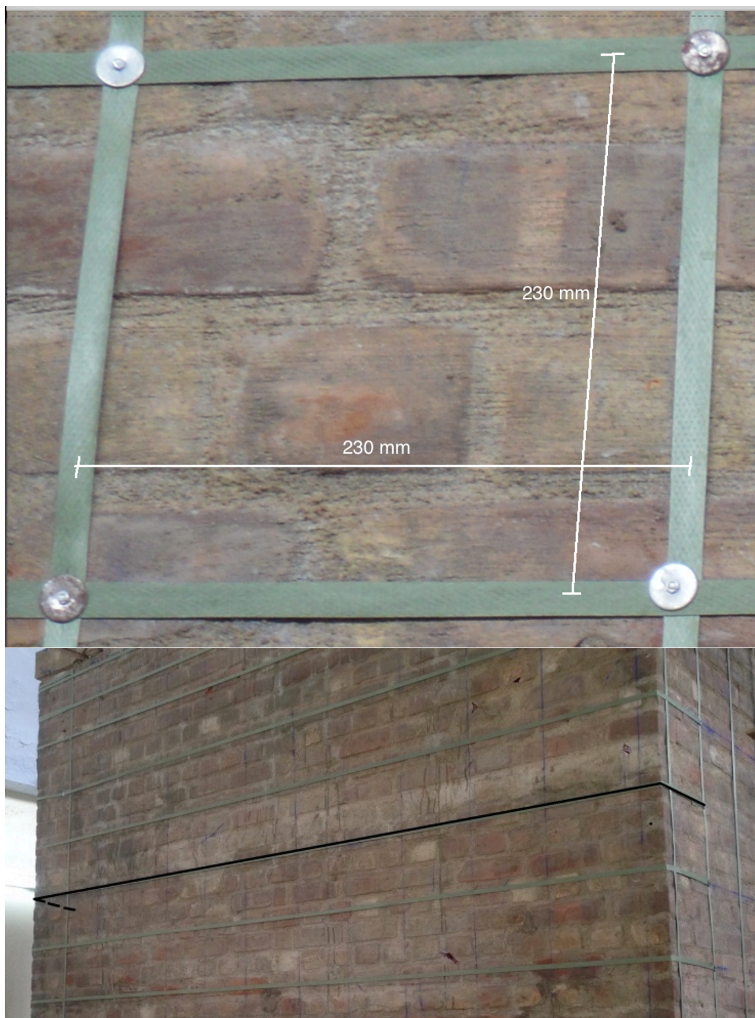
Figure 7.3: Connection detail between horizontal and vertical bands spaced at 230mm ( top ), typical length and arrangement of horizontal PP-bands ( bottom )
