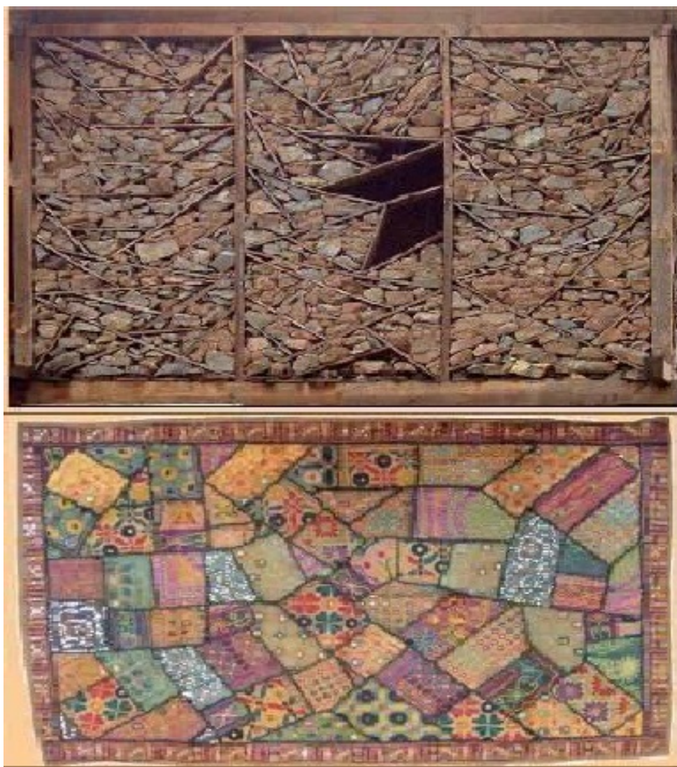
Figure 3.7: Dhajji Wall (Top), Patchwork quilt, 'Dhajji' in Persian [99]
