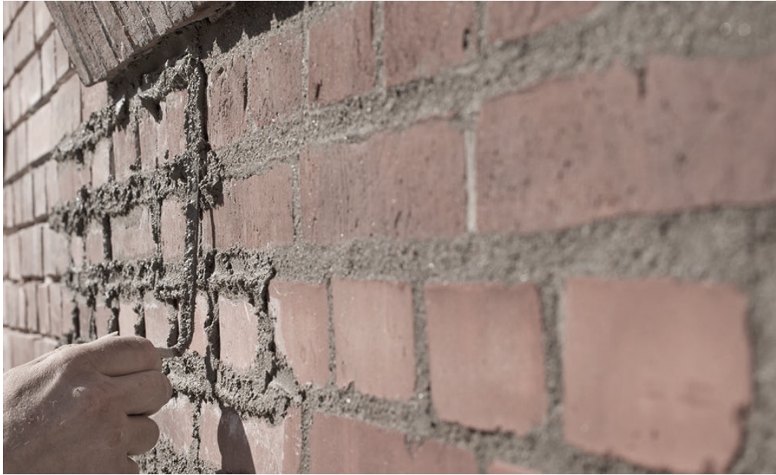
Figure 2.17: Re-pointing on brick masonry structure [54]
