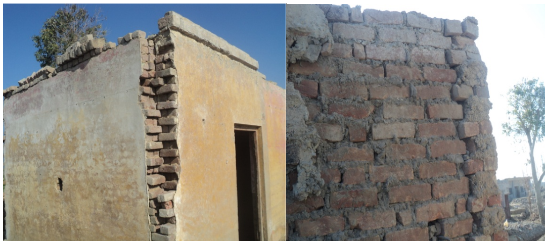
Figure 3.15: Poor Corner joints
