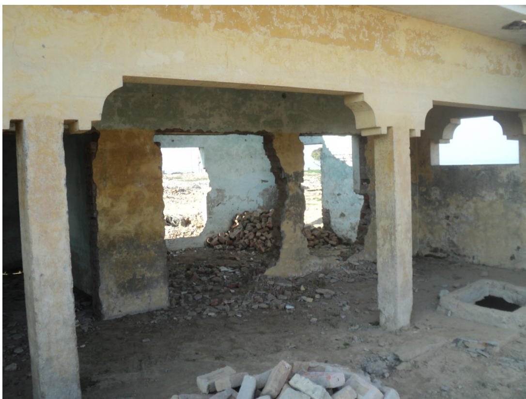
Figure 3.13: No consideration for opening size and location
