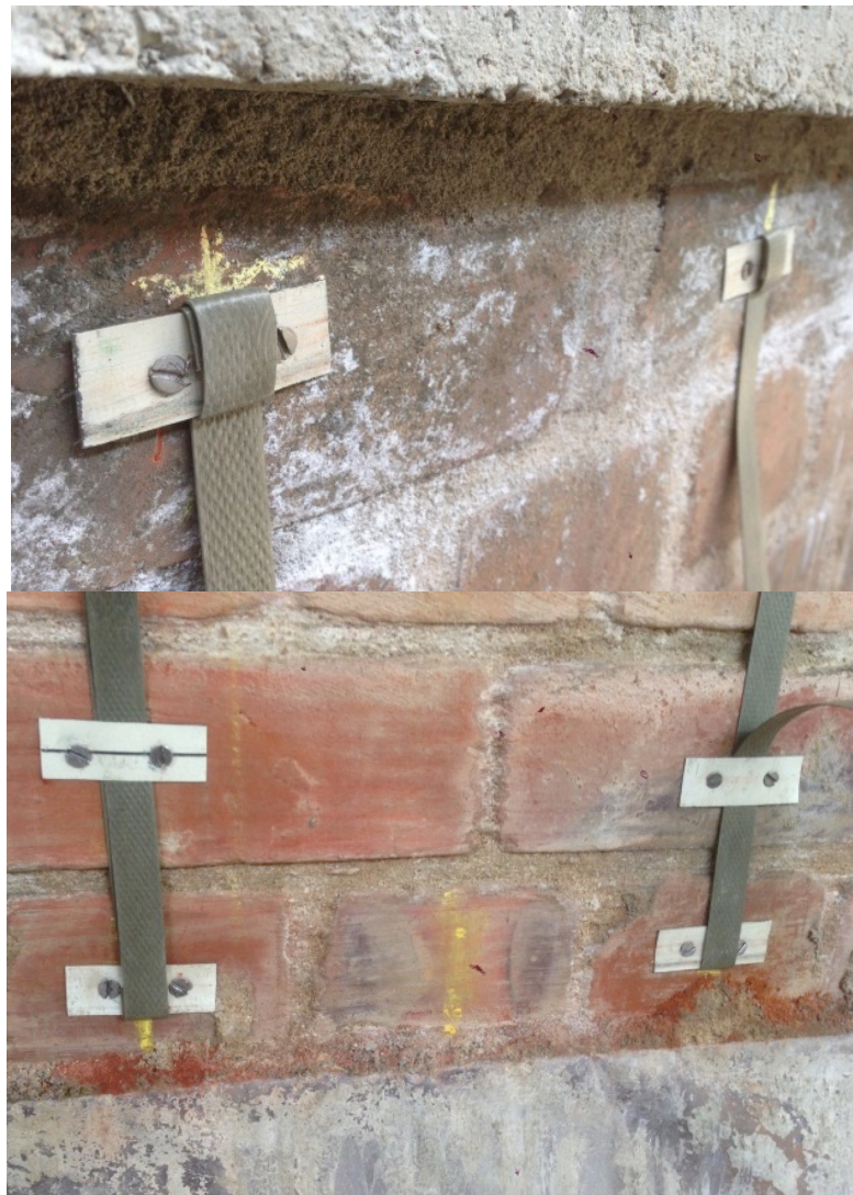
Figure 7.9: First end ( left ), Second end ( right ) revised connection detail for Room-2
