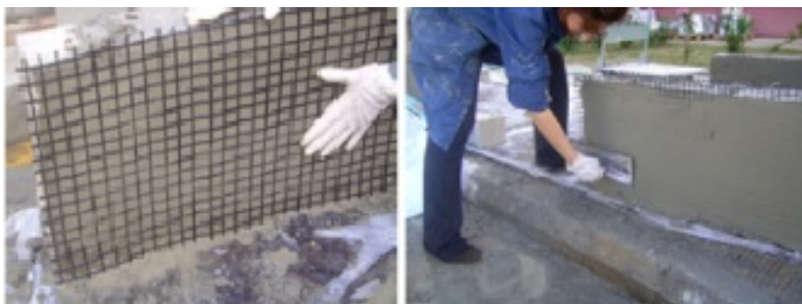
Figure 2.20: Application of Reinforcing mesh [60]
