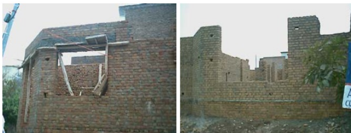
Figure 2.29: Discontinuous lintel band (left), Large window opening (right) [11]
