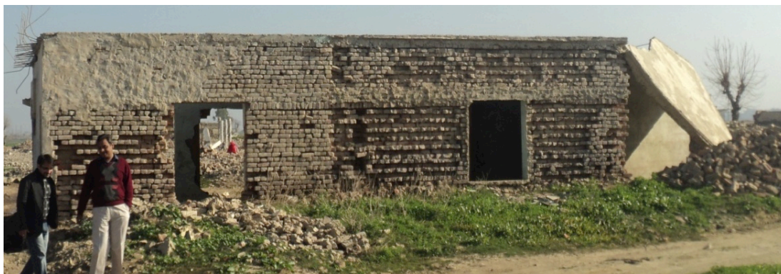
Figure 3.12: Absence of RCC lintels over openings
