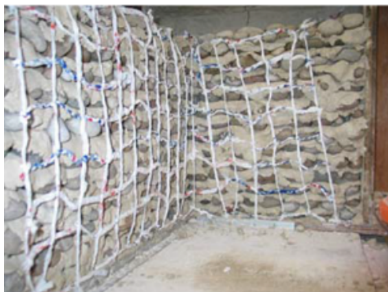
Figure 2.23: Plastic Carrier bag retrofit for masonry [75]
