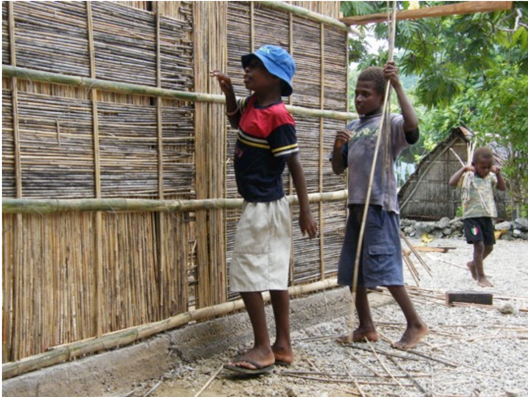
Figure 8 Children assist in construction of a cane house, one of few remaining kanayumā sits behind
