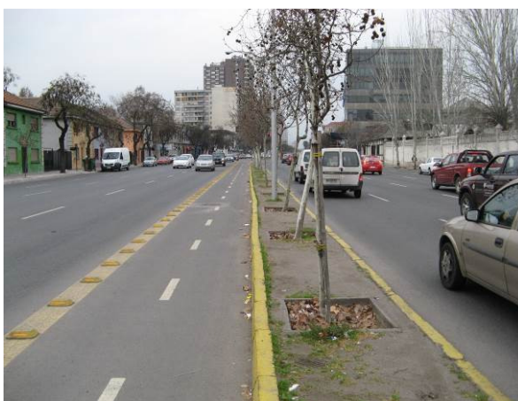
Figure 6-9: Cycle path on the carriageway adjacent to the central median. Blanco Encalada, Santiago, 24/08/2011. IMG_2419.
