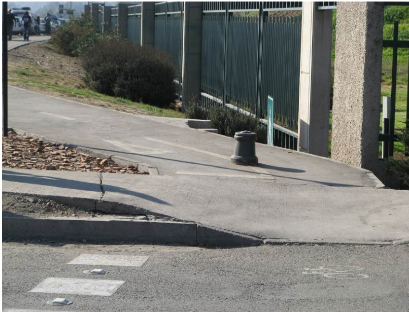
Figure 6-19: A bollard, a rather sharp curve and a steep curb cut require a considerable reduction in speed from the cyclist. Las Perdices, La Reina, 01/05/2011. IMG 2112.
