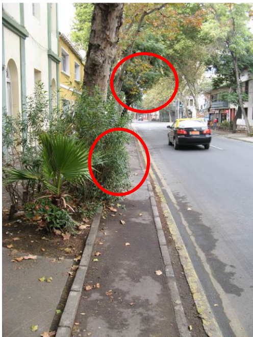
Figure 6-6: Bushes and low-hanging branches can be significant obstacles, especially when the cycleway is narrow. Club Hípico, Santiago, 23/04/2011. IMG_2062.
