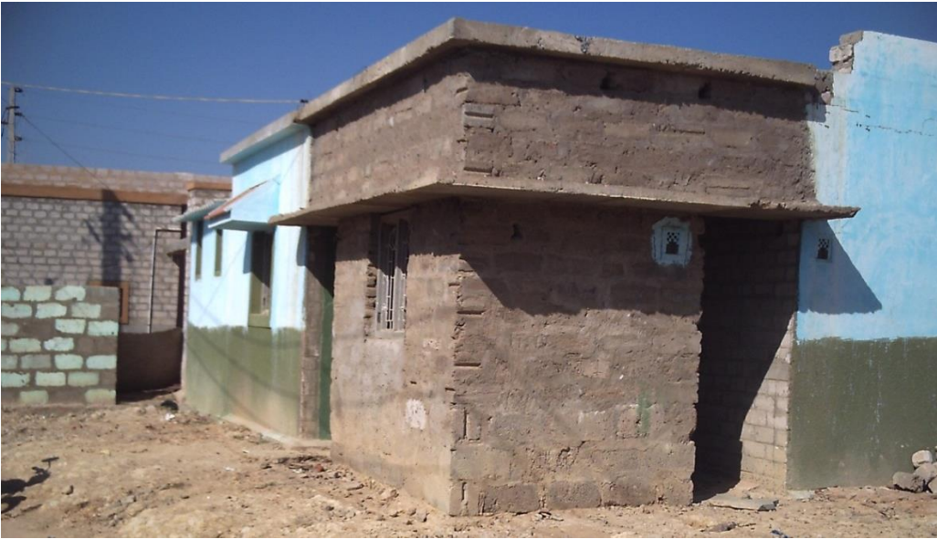
Fig. 4.28: Self-built infill construction to the open corner of a Hunnarshālā-designed cluster scheme, built using new materials (SRE block and reinforced concrete). An attempt at design continuity with the new house is evident, along with elements particular to traditional Kutchi houses, such as the small gokhals (niches) to either side of the main door.
