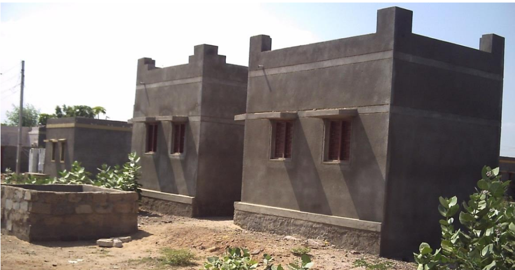
Fig. 4.29: Detached single dwellings incorporating the same elements as found in the cluster housing, but accommodating the new building regulations. The plinth, lintel and roof are emphasised in the rendering, speaking of the traditional salaat building process.
