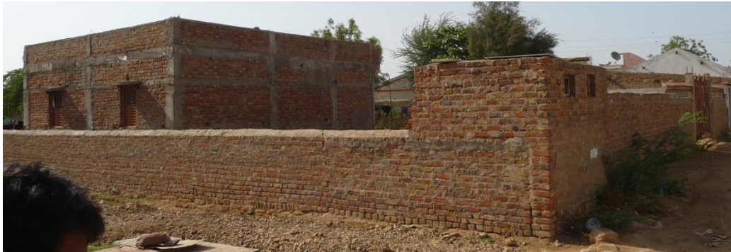
Fig. 4.69: A new house showing the new use of concrete reinforcement beams with customary clay blocks rather than SRE blocks as per Hunnarshālā's process. Nonetheless, the aesthetic is that of reconstructed house, as are certain features such as the projecting lintel-level window shades.
