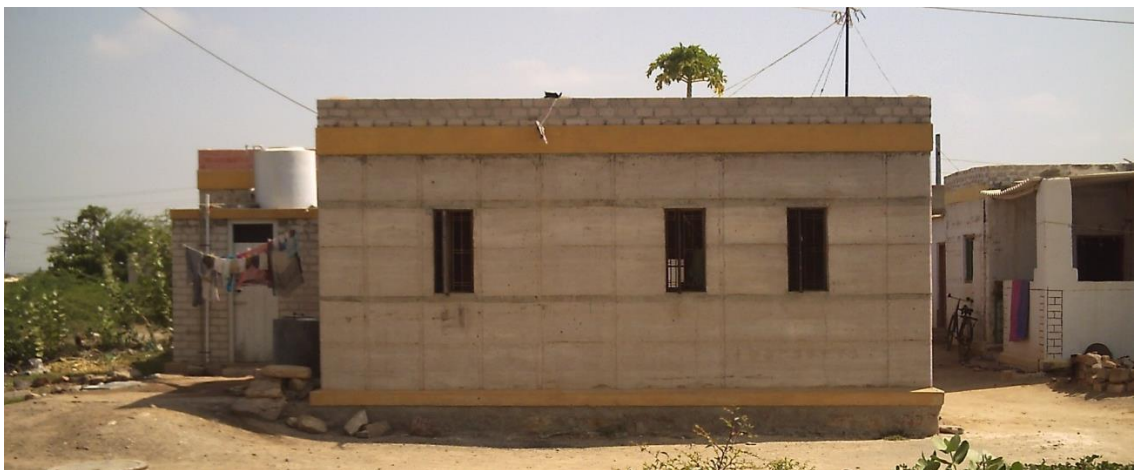
Fig. 4.34: Stabilised rammed-earth (light grey) with concrete ring beams (dark grey, yellow).
