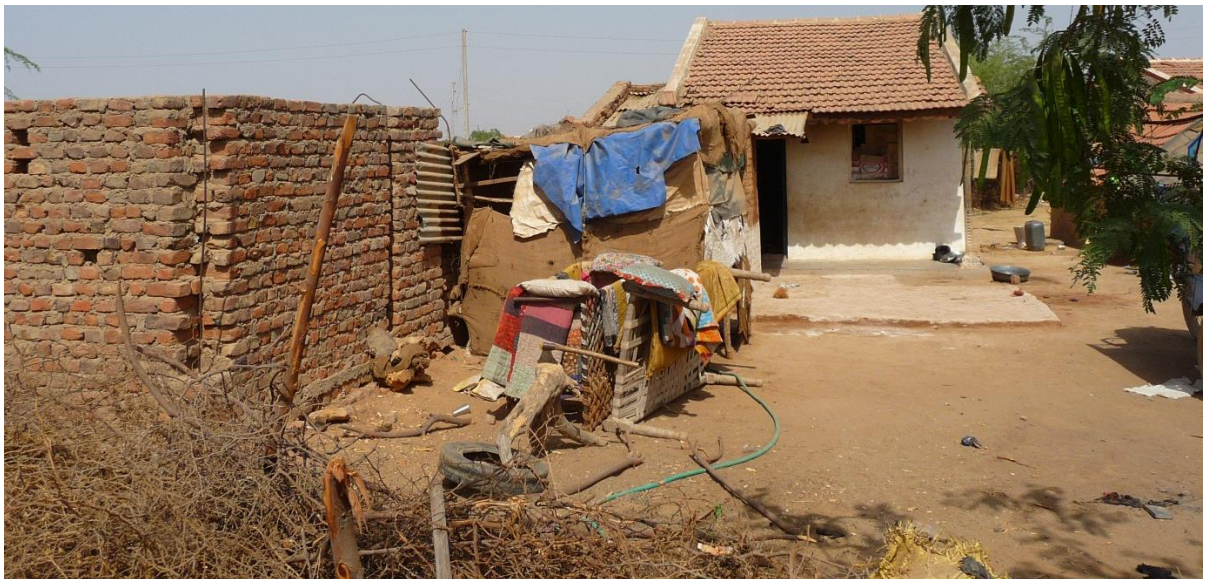
Fig. 4.63: House at Junawada showing donor house (white, tile roof) with subsequent informal additions, including a roofless brick-built building that will serve as a home for the family, and a tent-like structure linking the two, built from very basic, apparently 'found' materials. These structures often serve as kitchens and an eating spaces.
