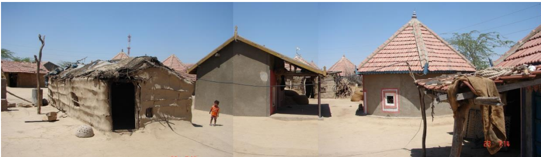
Fig. 4.49: New cluster around an as yet relatively undefined falia , with rectilinear and circular planned buildings. Note the retained original earth-constructed building (left foreground) which, despite its dilapidated condition, is still used and also the self-built chamod (right foreground), built of found materials, including Mangalore tiles.
