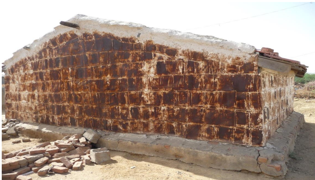
Fig. 5.3: Oil tin clad house, Junawada
