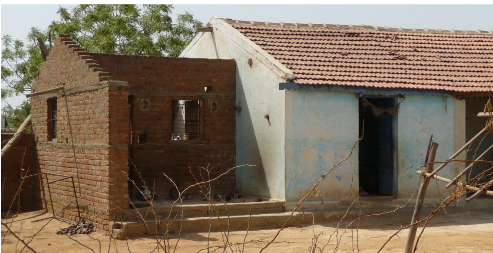
Fig. 4.71: A new extension to a reconstructed house which, although incomplete, is already used as a space for cooking. The raft foundation in the foreground implies on-going further development. Note that concrete ring-beam construction has been used, although stabilised rammed-earth blocks have been replaced by more traditional clay bricks.
