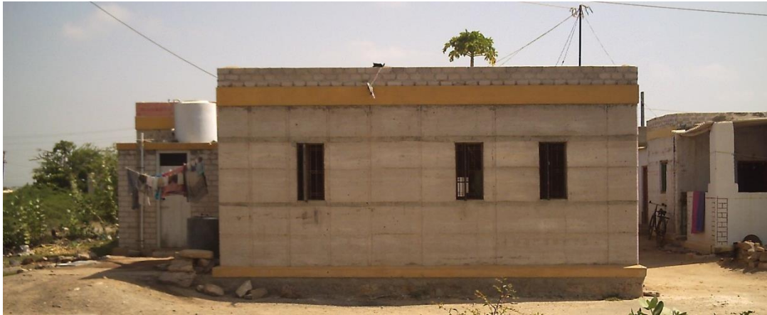
Fig. 4.30: An unfinished detached single dwelling, displaying the materiality of the stabilised rammed-earth construction.
