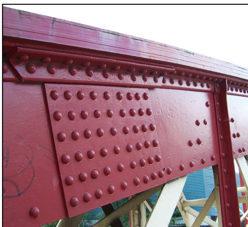
Figure 6.9 Side view of top chord of main girder. Extensive riveting was employed to fix the 7 layers of plate iron of the top chord flange. (Photos by M.O'Sullivan 2008)
