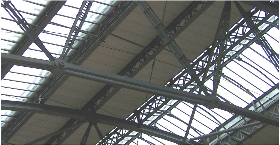
Figure 8.7 Bottom chord of Liverpool Lime Street Station roof truss (O'Sullivan 2009)
