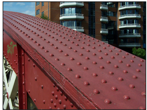
Figure 6.5 Side view of top chord of main girder. Figure 6.6 View of top chord. No sign of inter-plate rusting. Some edge rusting is visible in Figure 2.6 (Photographs by M.O'Sullivan 2008)
