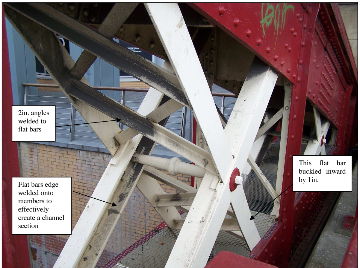
Figure 6.19 Strengthened members of the bow-string girder. (Photo by M. O'Sullivan 2008)
