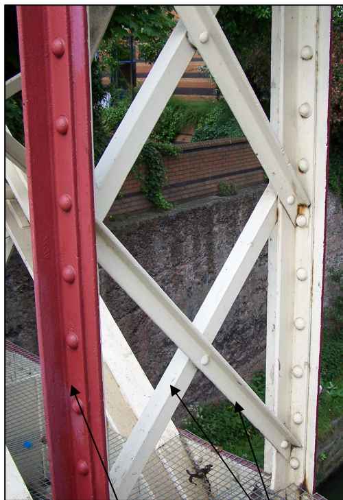
Figure 6.11 Connection of vertical strut and diagonal ties to inside of upper chord web. (Photo by M.O'Sullivan 2008)
