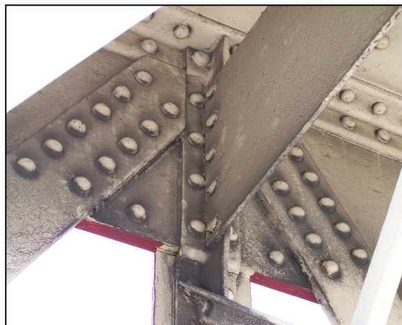
Figure 6.11 Connection of vertical strut and diagonal ties to inside of upper chord web. (Photo by M.O'Sullivan 2008)
