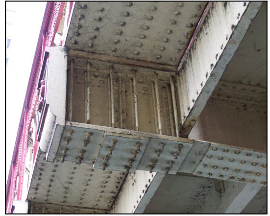
Figure 6.16 View of cross girder connection from below (Photo by M O'Sullivan 2008)
