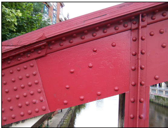
Figure 6.5 Side view of top chord of main girder. Figure 6.6 View of top chord. No sign of inter-plate rusting. Some edge rusting is visible in Figure 2.6 (Photographs by M.O'Sullivan 2008)
