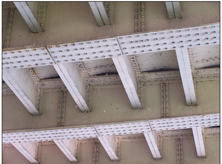
Figure 6.17 Underside of road deck showing curved buckle plates. (Photo by M. O'Sullivan 2008)
