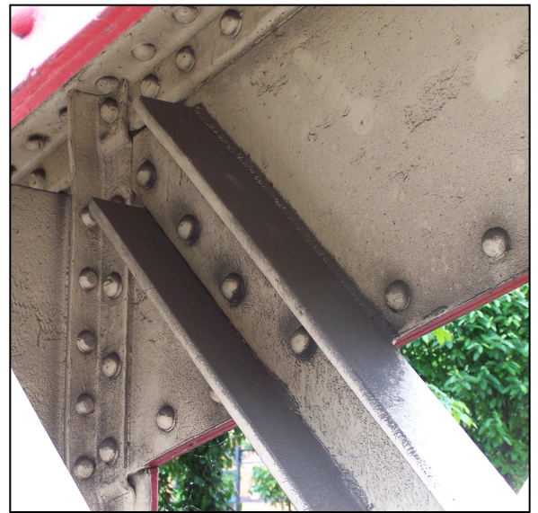
Figure 6.21 Tie-bar strengthened by creating a channel section. (Photo by M.O'Sullivan 2008)
