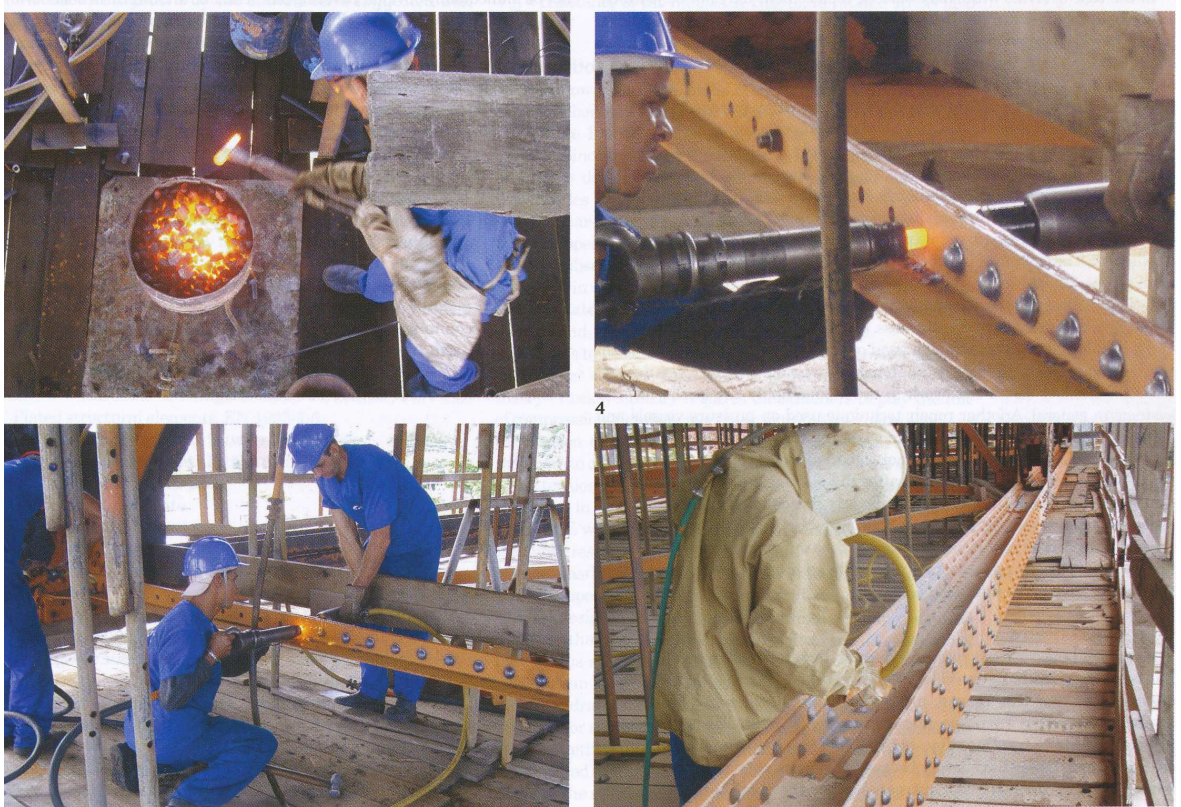
Figure 4.31 Steel riveting operation in the refurbishment of Hercilio Luz Bridge, Brazil (Lamb 2008).
