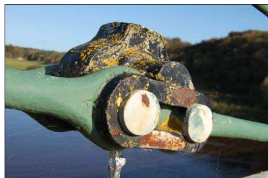
Figure 1.26 Coupling link in suspension chain of Union Bridge (Photo from bbc.co.uk accessed July 2012)
