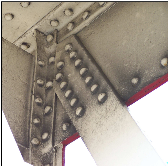
Figure 6.20 Typical tie-bar to upper chord connection. (Photo by M.O'Sullivan 2008)
