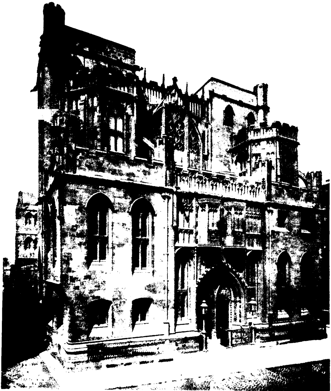
EXTERIOR VIEW OF THE LIBRARY .
