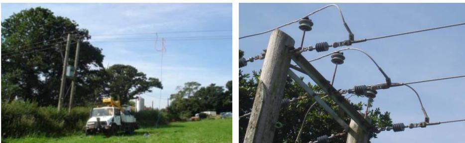
Figure 5.11 Detail of the connections of Circuit IV recovered insulators
