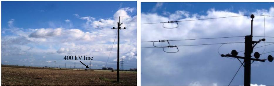
Figure 5.8 Detail of the connections of Circuit I recovered insulators
