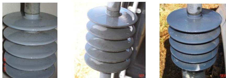
Figure 5.26 View of the Circuit I insulators after spraying to see hydrophobicity classification. Both sides have the same condition (HC7)
