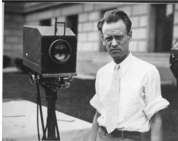
Figure 4.11 Philo T Farnsworth and image dissector camera (head only, a very large amount of external electronics was also needed). Date: about 1934. Picture source: Kent Farnsworth http://www.philotfarnsworth.com Accessed 11/06/2006
