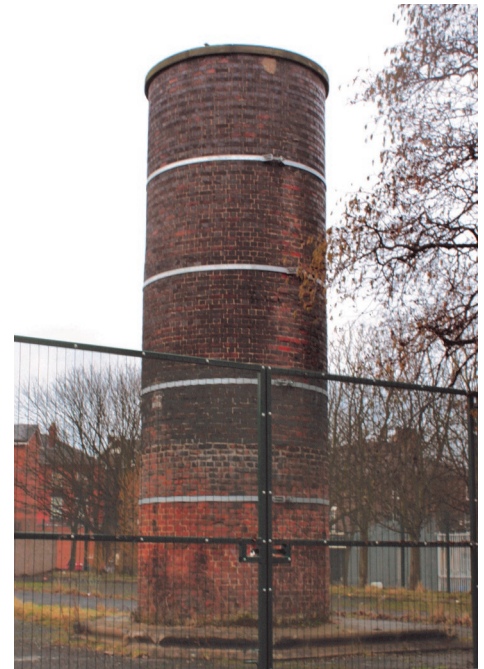
Figure 10: Ventilation shaft for the Victoria tunnel, Shenstone Street.
